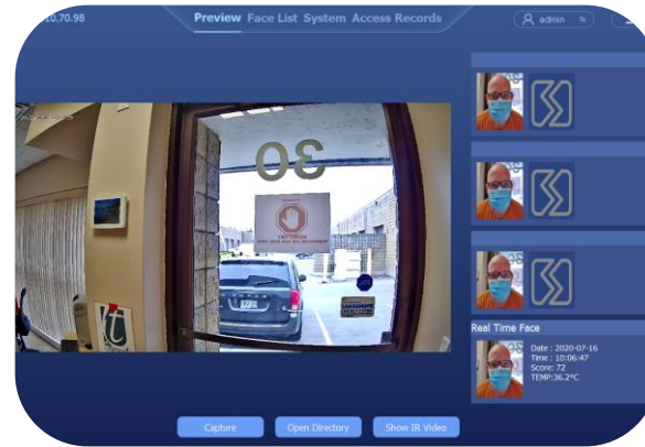
Remote viewer installed on reception/security computer
